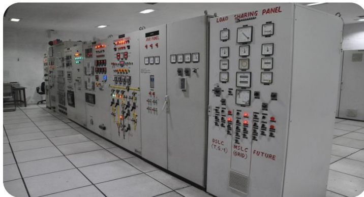
Cogeneration Control Panel
