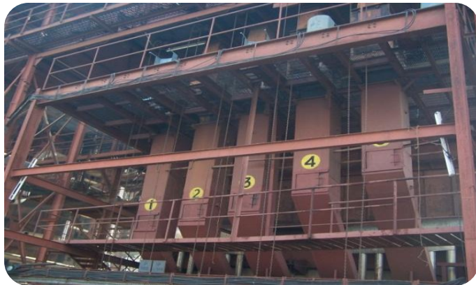
Bagasse Silos & Feeders of Boiler
