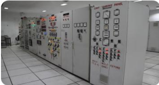
Cogeneration Control Panel
