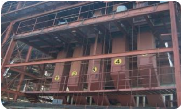
Bagasse Silos & Feeders of Boiler
