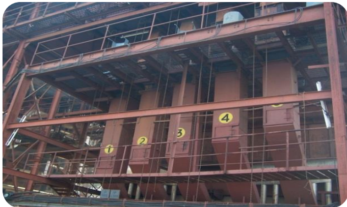
Bagasse Silos & Feeders of Boiler
