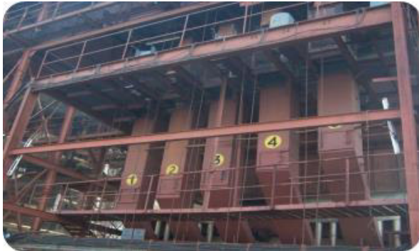
Bagasse Silos & Feeders of Boiler
