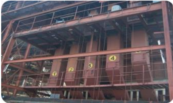
Bagasse Silos & Feeders of Boiler
