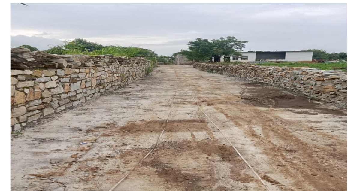
Construction of CC Road at village
