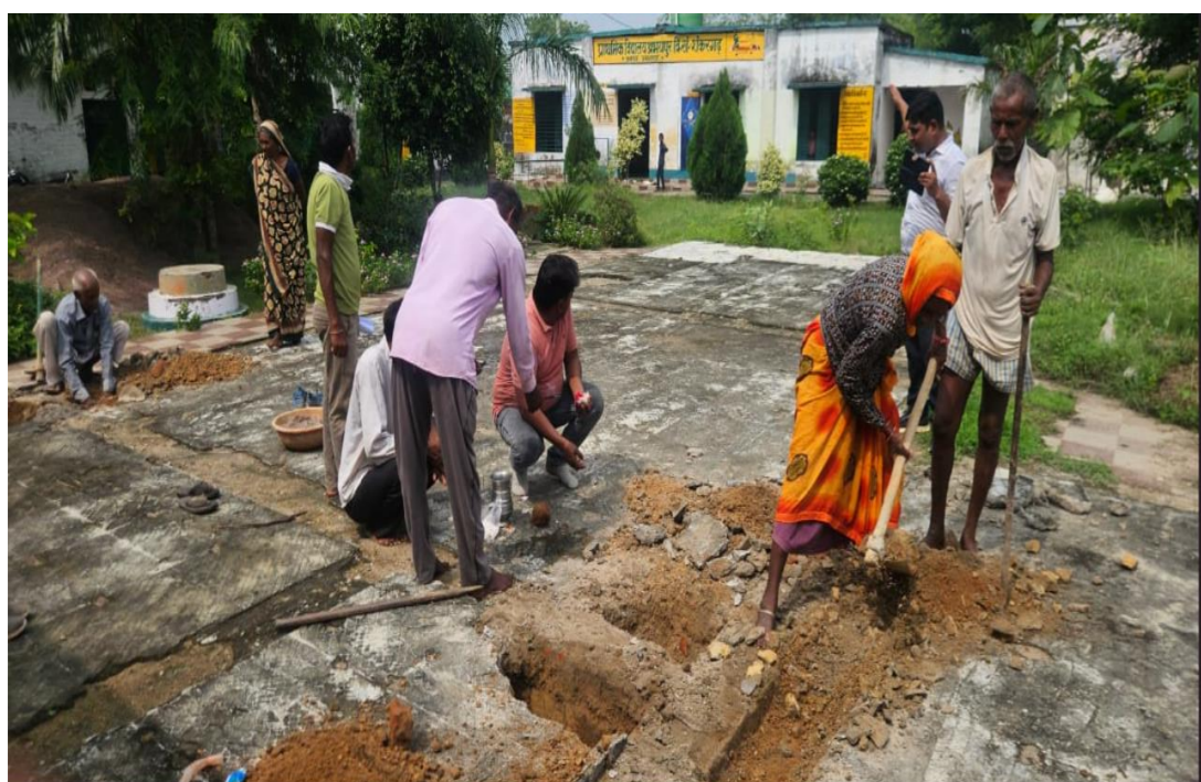
Renovation of Primary School
