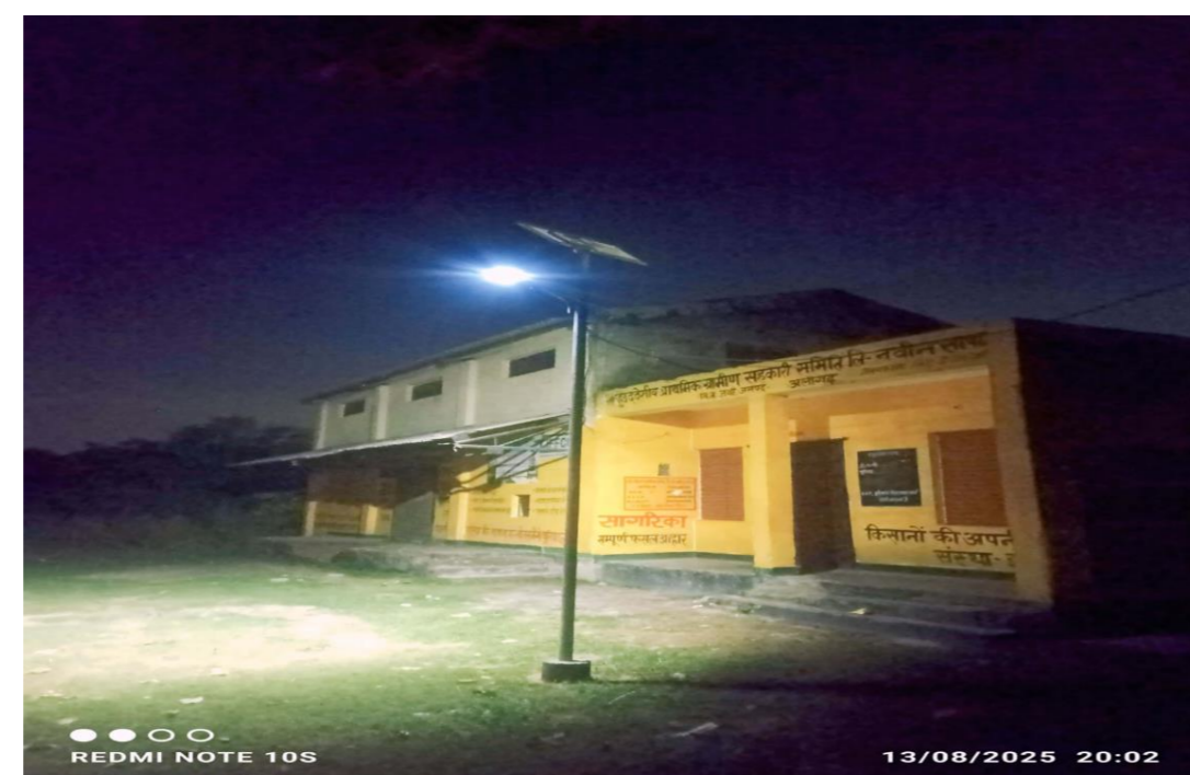
Solar Light Installation
