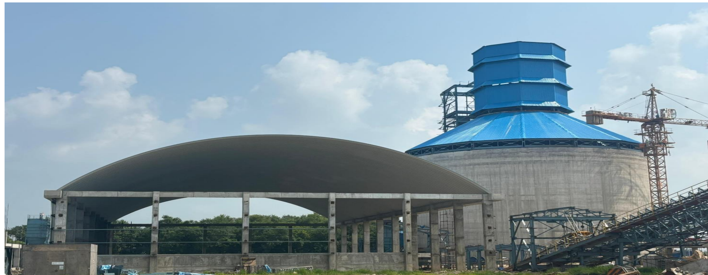
Additive Shed & Clinker Silo
