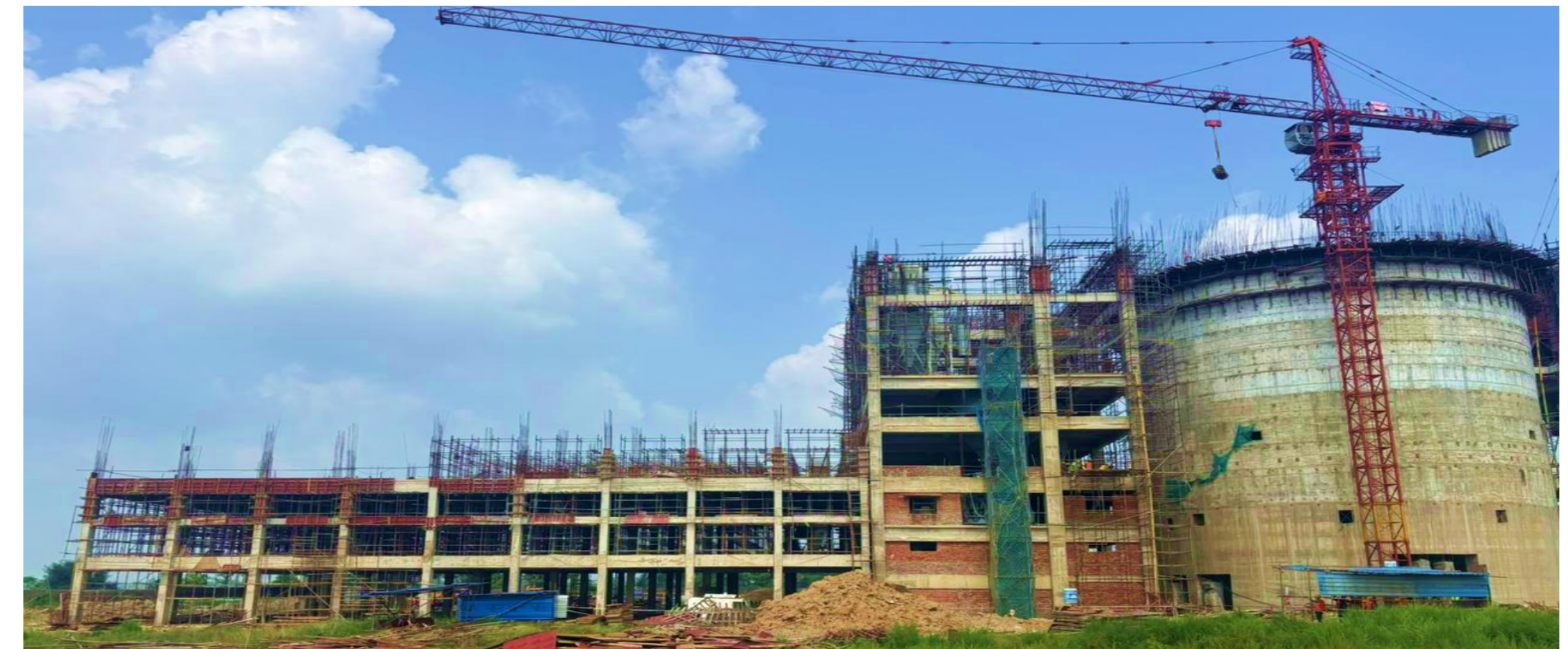
Packing Plant Building & Cement Silo
