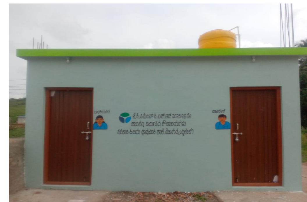
Construction of Toilet at School
