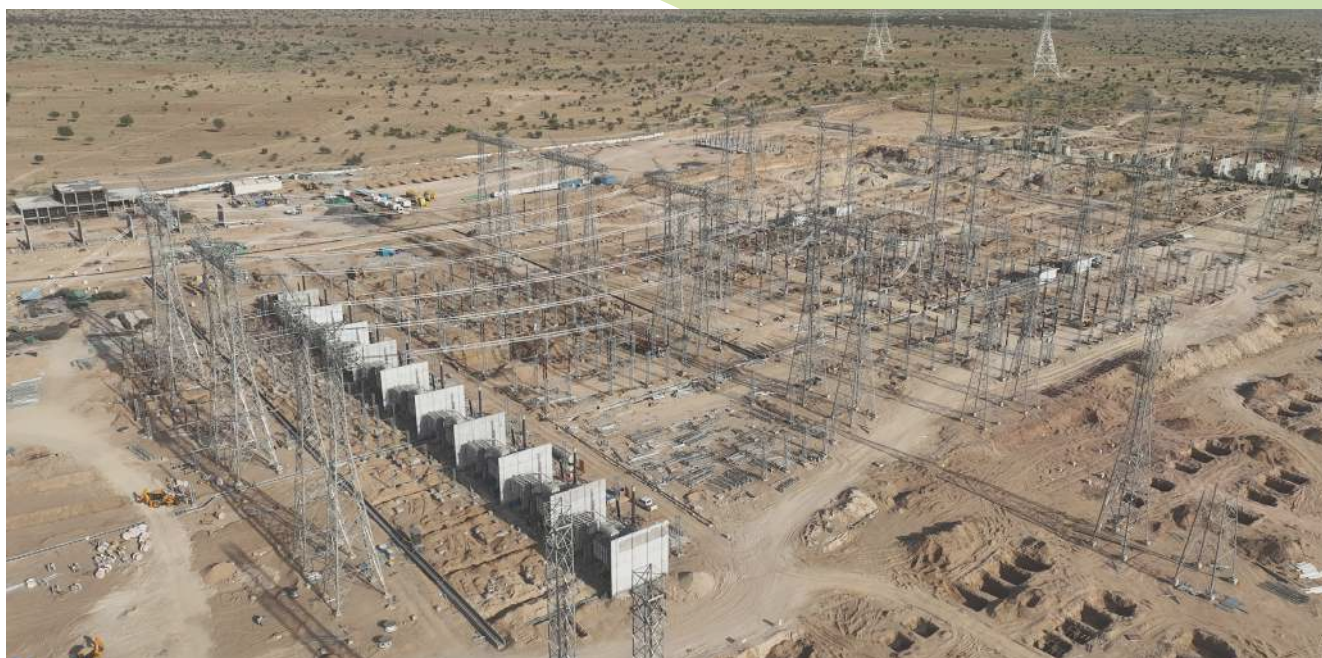
Air Insulated Substation (AIS) work in progress at Fatehgarh, near Jaisalmer, Rajasthan
