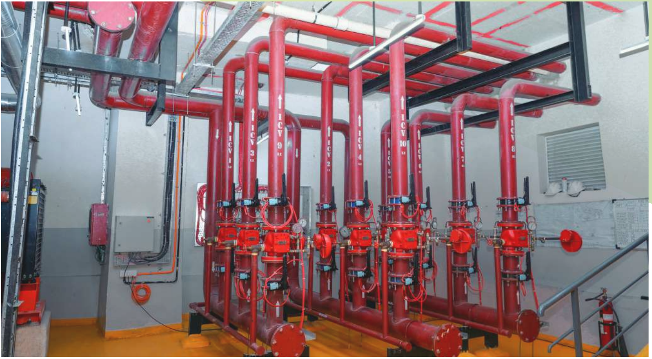
Firefighting work at Phoenix Centaurus, Hyderabad
