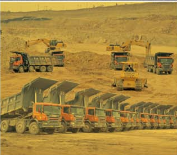
Rohtak-Panipat Section of NH-17a : work in progress
