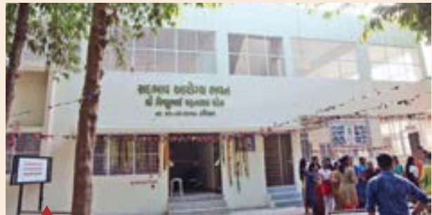
New Construction at M. B. Patel Trust Hospital
