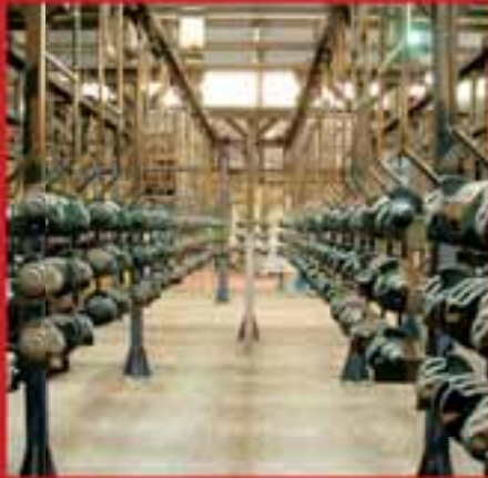
CRANKSHAFT FACILITY AT CIE FORGINGS GALFOR, SPAIN
