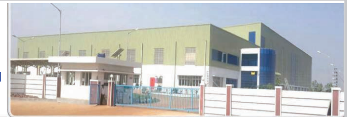
New Stampings Plant at Zaheerabad
