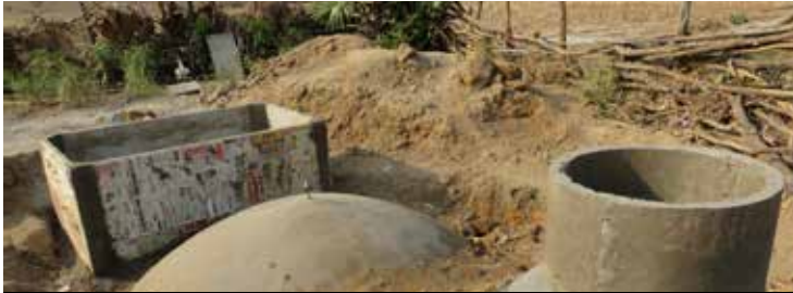
Waste management through bio-digesters. Using cattle waste to provide biogas to rural homes. Hence reducing smoke pollution, methane & dependency on firewood, Adilabad, Telangana
