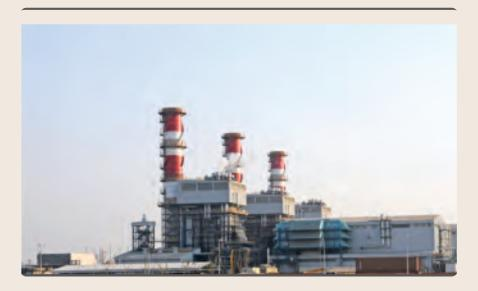
GEN- the 1200 MW Greenfield gas based power generation Plant has in-built efficiency enhancing design features and state of the art technology. The single shaft configuration saves on the length of steam cycle piping and requirement of major operating equipments; thus enhancing the throughput. Special metallurgy of vanes and blades, matching triple pressure heat recovery steam generator, special hydraulically controlled axial positioning device and advanced design fuel burners
