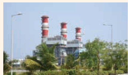
DGEN Power Plant
