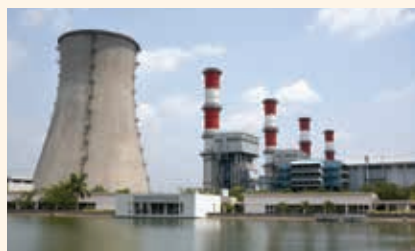
SUGEN Power Plant
