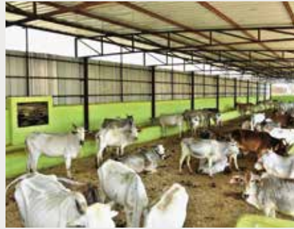
Constructing sheds for animal welfare
