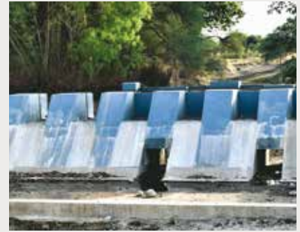
Construction of the Anicut Dam for irrigation
