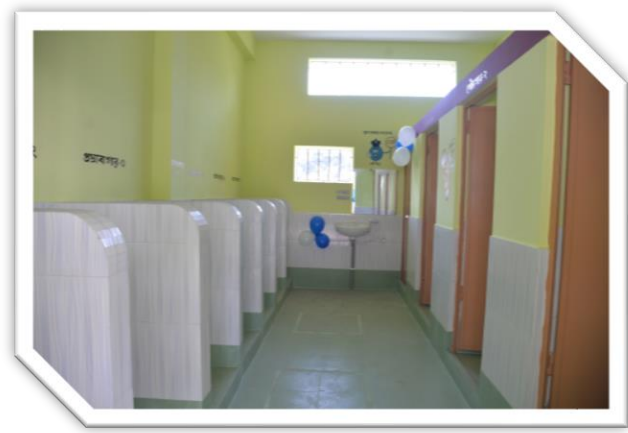
Toilets Constructed in Schools- West Bengal & Haryana
