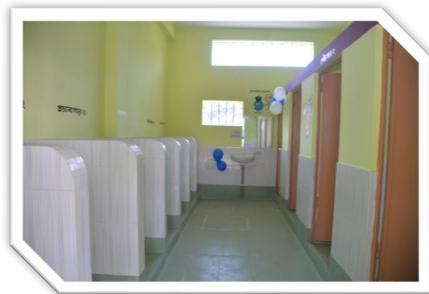
Toilets Constructed in Schools- West Bengal & Haryana
