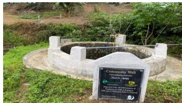
Well Restoration – Kalvarayan * Jawadhu Hills
