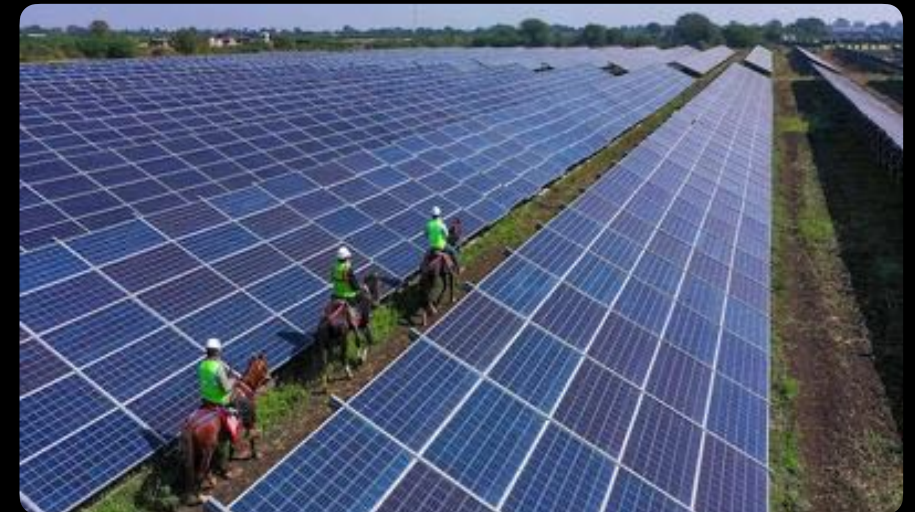
Pictures depicting the commissioning of the solar power project
