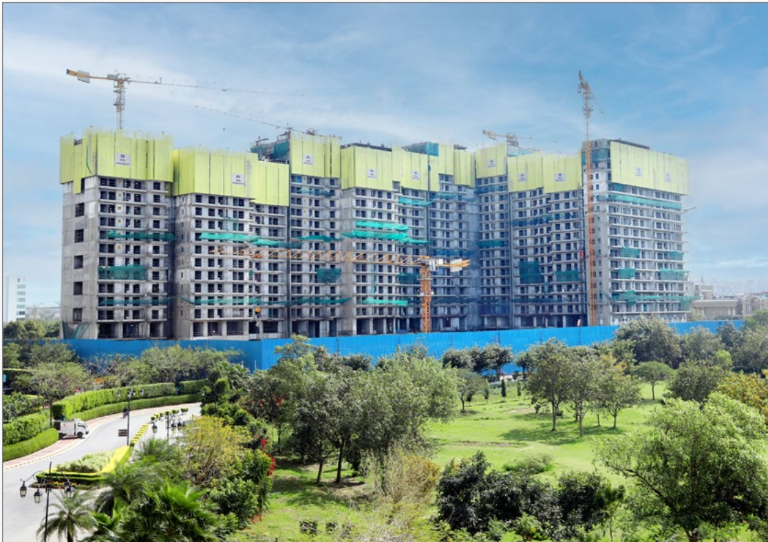
ONE Midtown under construction in New Delhi
