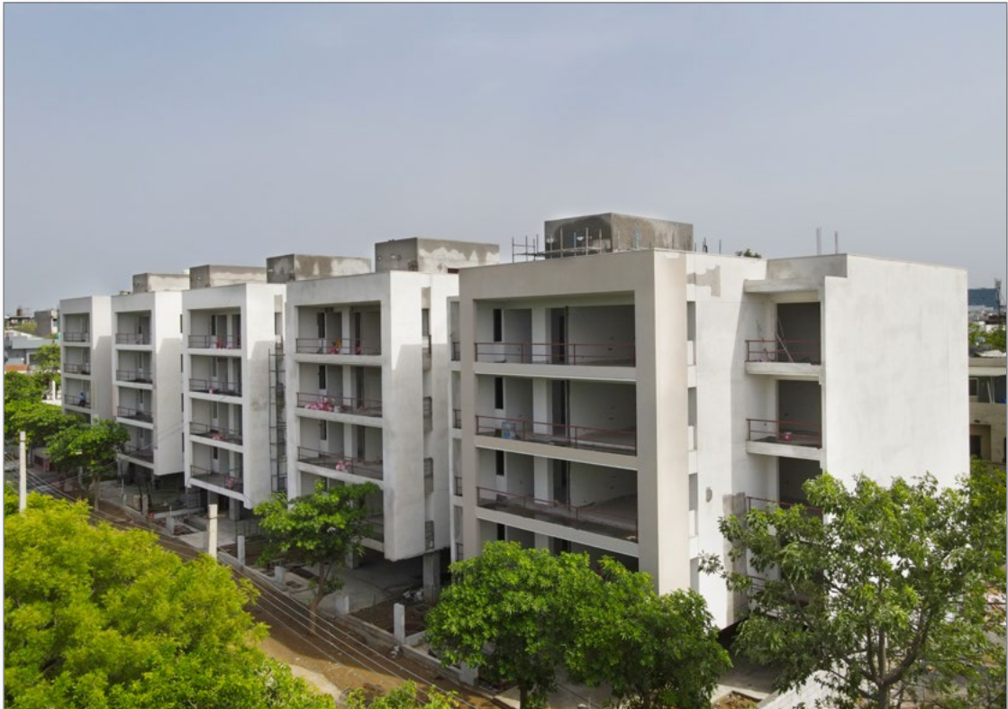
Mousari Enclave under construction in DLF City Phase III, Gurugram
