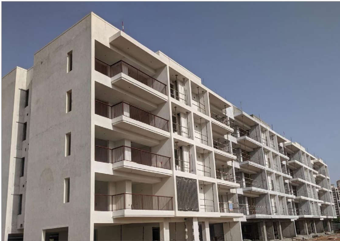
Independent Floors at Garden City under construction in Sectors 91/92, Gurugram
