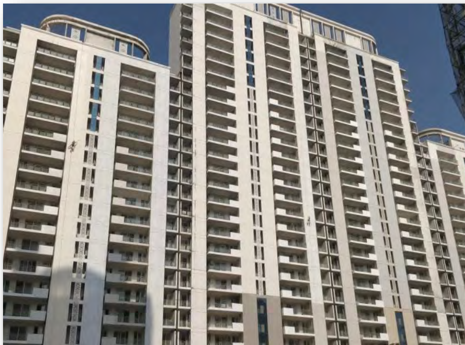
Ultima, Gurugram (Under construction): 0.31 msf
