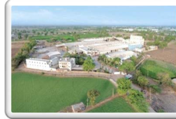
AGL Idar Plant (Floor Tiles)
