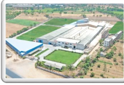
Amazone Dalpur Plant (Floor Tiles)
