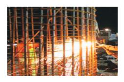
The welding performance is an important indicator of TMT bar. After welding, the microstructure and properties of the weld and heat affected area will change and become weak point of the bar. The amount of carbon content in steel has been a major deciding factor and an excess of carbon content threatens, its property of weldability. Simhadri TMT steel bar with low carbon content has In-built ability to resist loss of strength at high temperature, can be butt welded & lap-welded.
