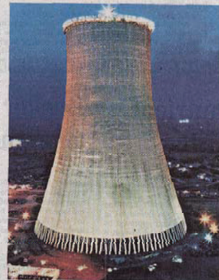
Natural draft cooling tower at the Kalsindh power plant of Rajasthan Rashtriya Utpadan Nigam Ltd. in Rajasthan, claimed to be the world's tallest (202 metres). — PHOTO: HANDOUT/EMIL
