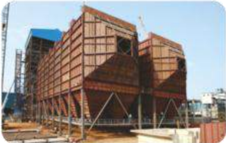
AIR POLLUTION CONTROL EQUIPMENT
