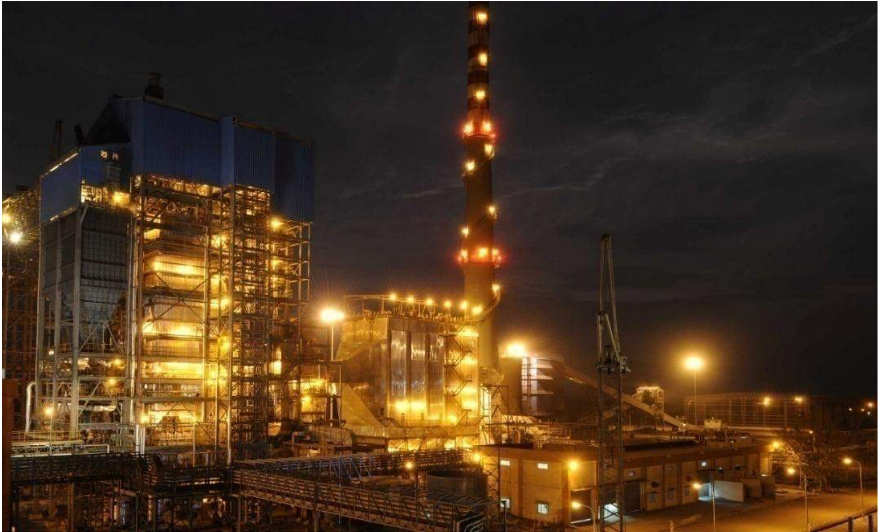
45 MW Power Plant with 1 x 190 TPH, 110 kg/cm 2 (g), 540 ± 5 Deg.C CFBC Boiler
