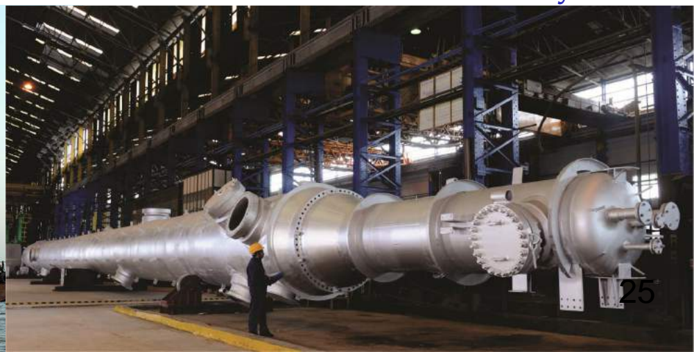
CCR Reactor under assembly
