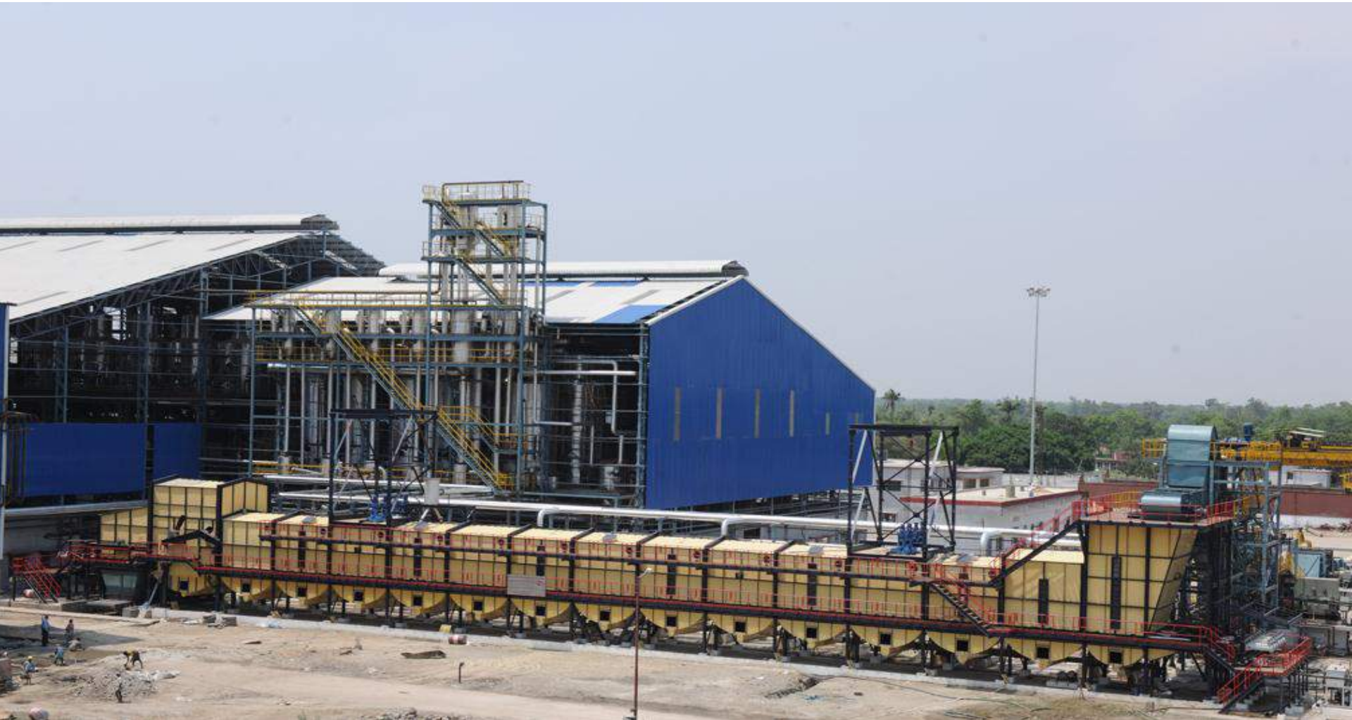
Chainless Cane Diffuser of 3500 TCD capacity
