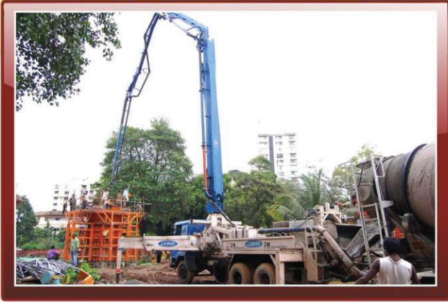
Concrete Boom Placer
