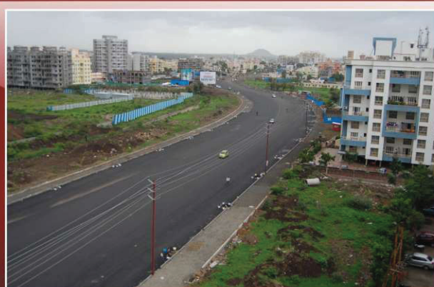
Kaspate Vasti, Pune Road
