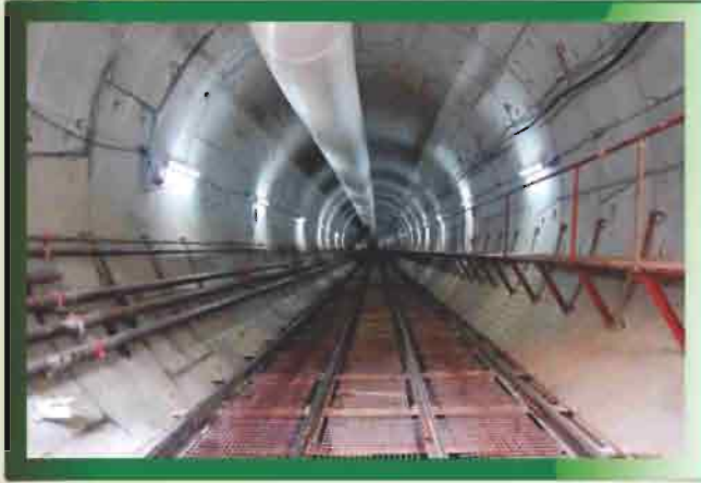
DMRC - Tunnel Projects
