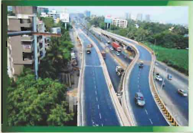
Amar Mahal Flyover
