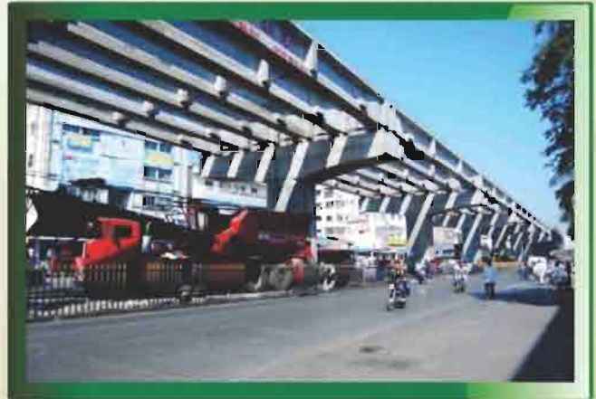
Dhankawdi Flyover Pune
