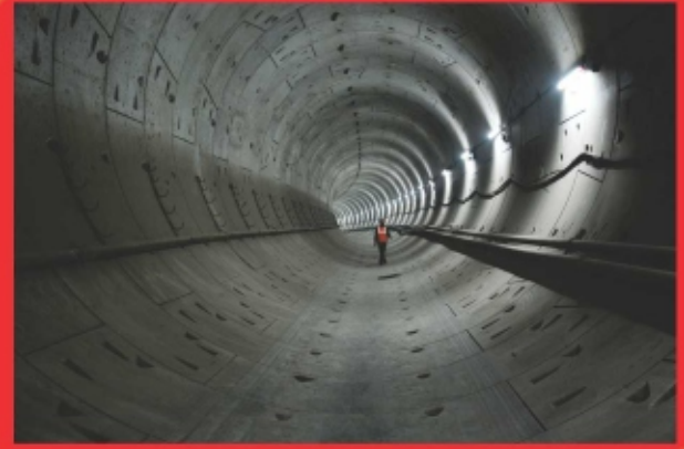
Delhi Metro Tunnel
