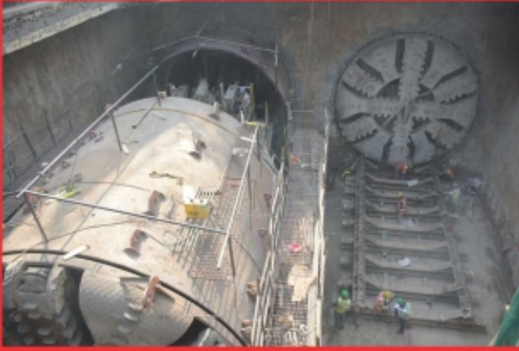
Underground Metro CC - 24
