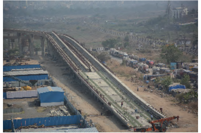
Navi Mumbai Metro Siding
