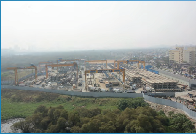
Malwani Casting Yard
