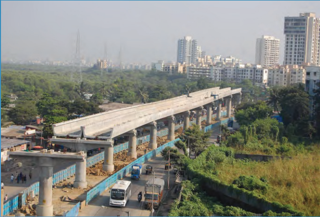
Mumbai Metro Line 2
