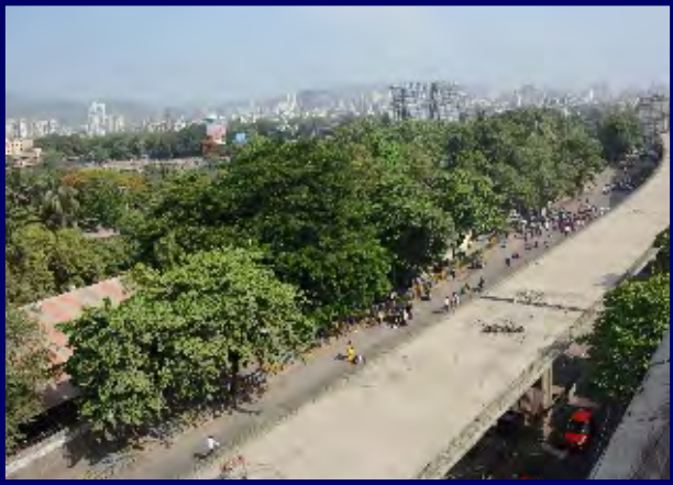
Kalwa Creek Bridge
