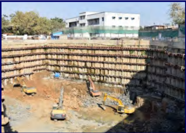
Sahar Metro Station at Mumbai
