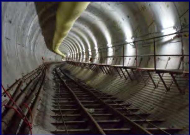
Tunnel From BKC to Vidyanagri
