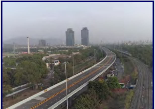
Ghansoli Flyover Navi Mumbai
