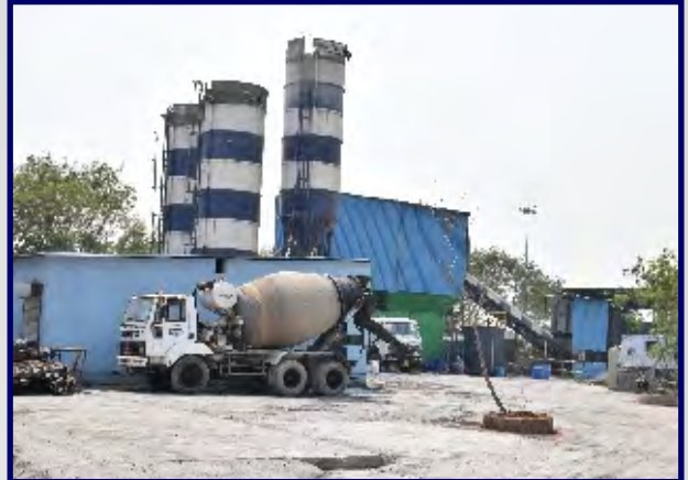
Ready Mix Concrete Plant
