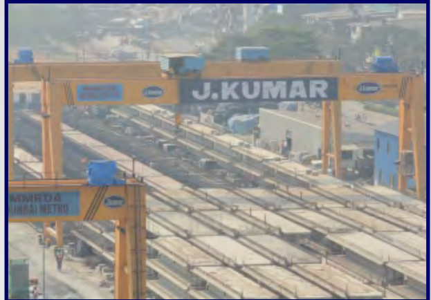
Girders for Elevated Metro
