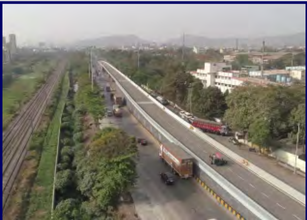
Thane Belapur Flyover
