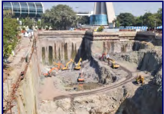
Domestic Airport Metro Station, Mumbai
