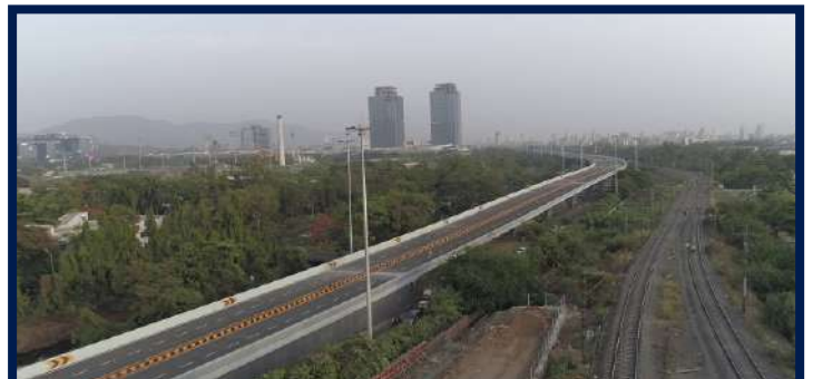
Thane Belapur Flyover
