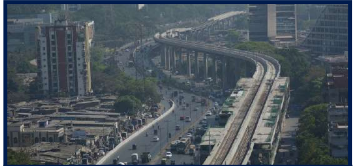
Mumbai Metro - Line 7
