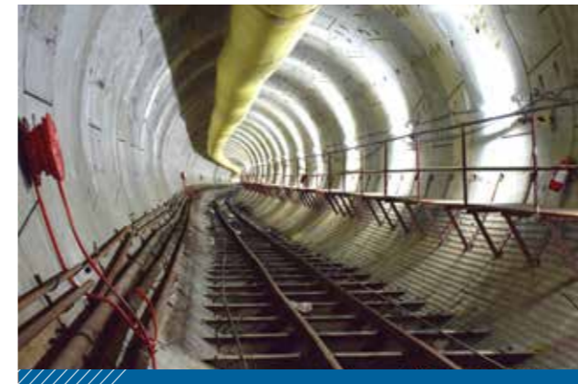
Mumbai Metro Line 3 Package 5 (BKC-Vidyanagri - Up line)
