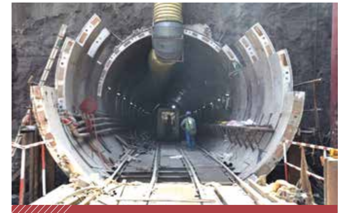
Mumbai Metro Line 3 Package 6
