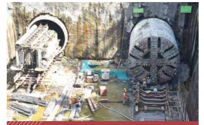
Mumbai Metro Line 3 Package 5 Vidyanagri South Retrieval Shaft
