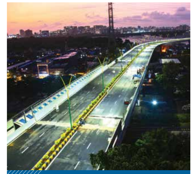
BKC- Chunabhatti Flyover
