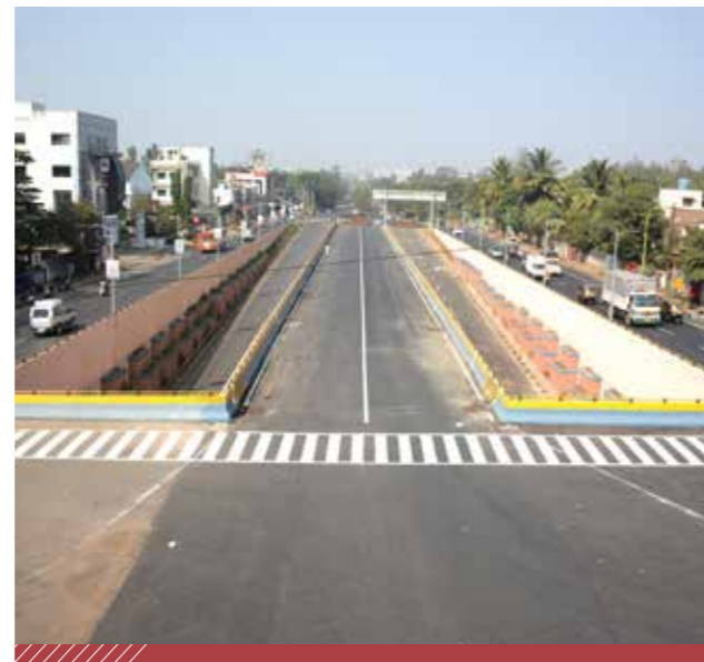
KSB Underpass, Pune
