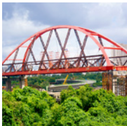
Kalwa Bridge Thane
