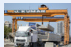
Casting yard (Elevated metro)
