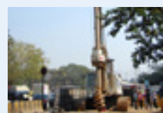
Hydraulic piling rig
