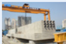
Casting yard (Underground metro)
