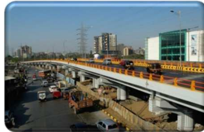
Flyover at Dindoshi, Mumbai
