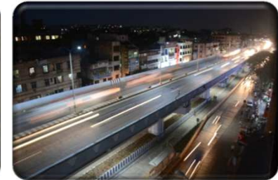
Flyover at Dhanakwadi
