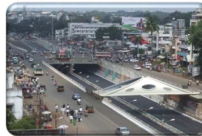
Grade Separator, Pune
