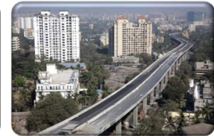
Flyover at Panjarapole, Mumbai
