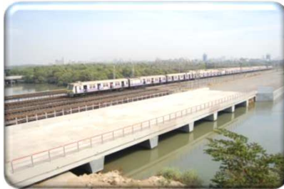
Bridge at Bandra -Mahim
