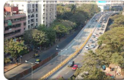
Flyover at Hindmata
