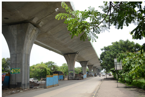
Thane Belapur Flyover
