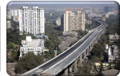
Flyover at Panjarapole, Mumbai
