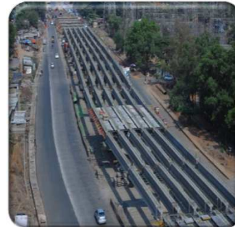
Mahape Flyover, Mumbai
