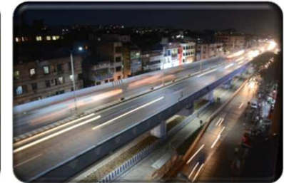
Flyover at Dhanakwadi
