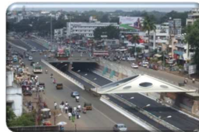
Grade Separator, Pune
