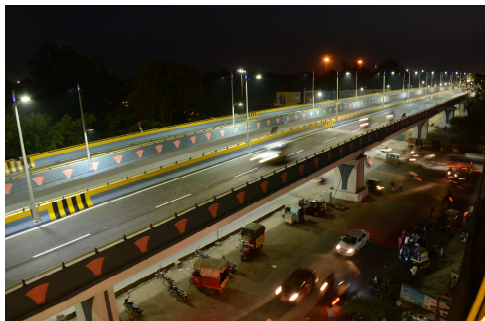
KSB Chowk Flyover, Pune
