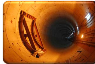
DMRC CC-24 Tunnel
