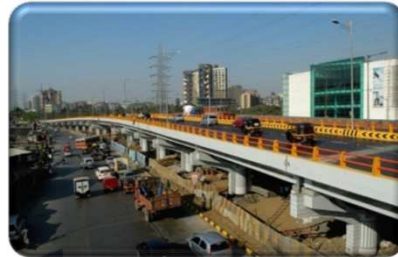
Flyover at Dindoshi, Mumbai
