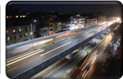
Flyover at Dhanakwadi
