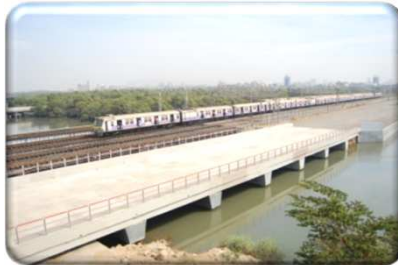
Bridge at Bandra -Mahim
