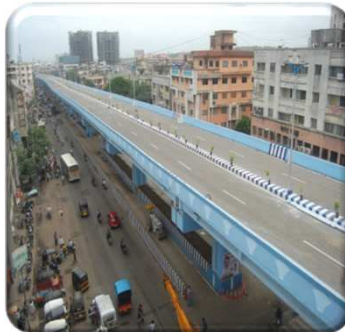
Dhankawadi Flyover, Pune
