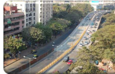
Flyover at Hindmata
