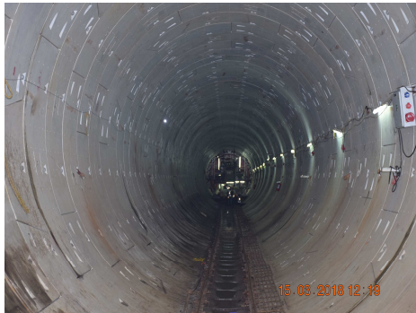
Mumbai Metro Line - 03
