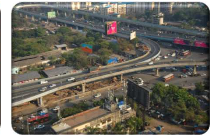
Flyover at Kapurbawadi
