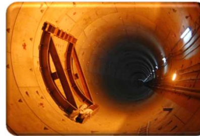
DMRC CC-24 Tunnel
