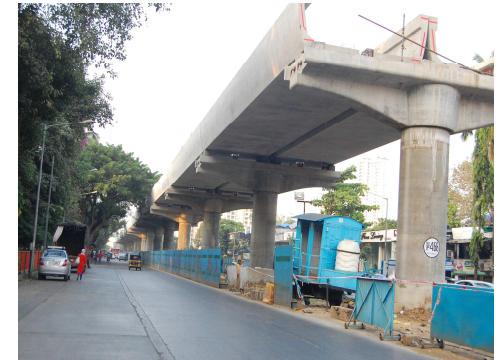
Mumbai Metro Line - 02
