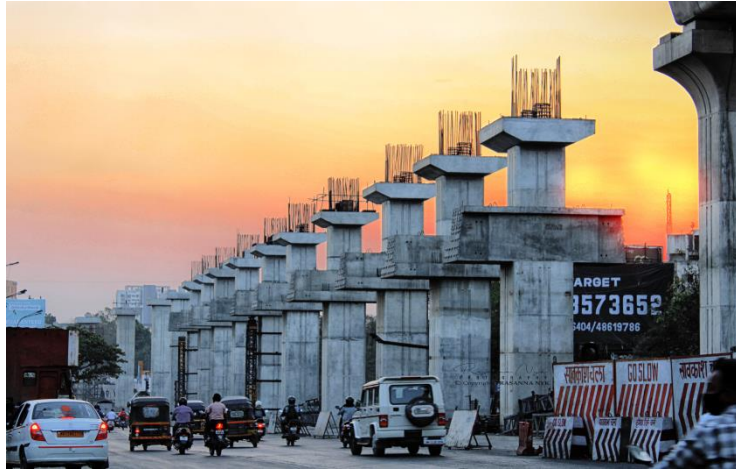
Pune Elevated Metro
