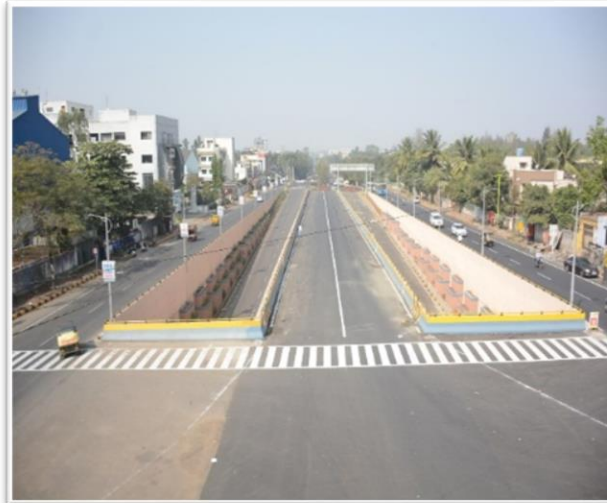
KSB Underpass, Pune
