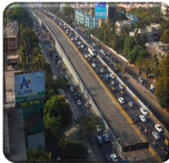
Kherwadi Flyover, Mumbai
