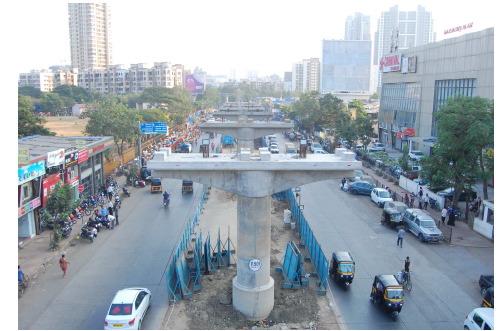
Mumbai Metro Line - 02
