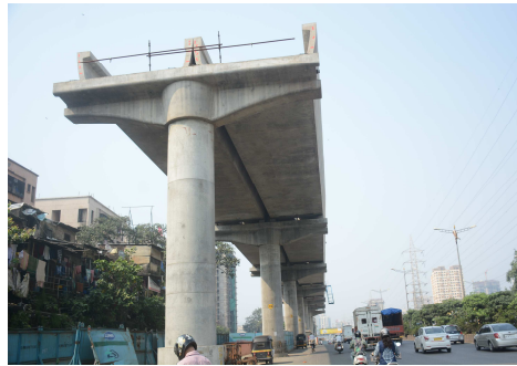
Mumbai Metro Line - 07
