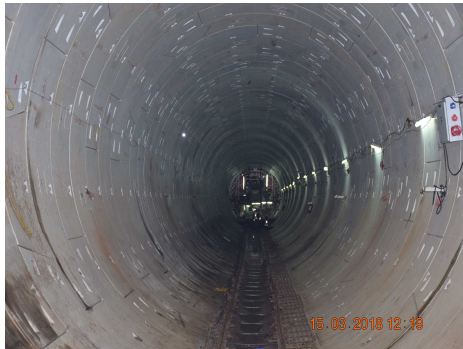
Mumbai Metro Line - 03
