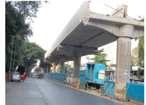
Mumbai Metro Line - 02
