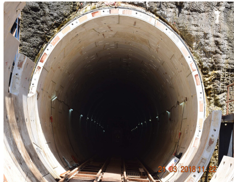
Mumbai Metro Line - 03
