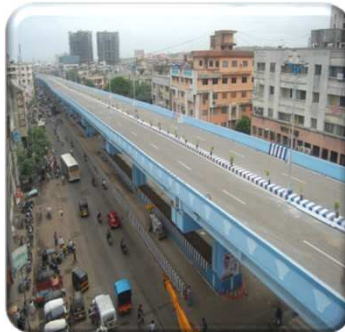
Dhankawadi Flyover, Pune
