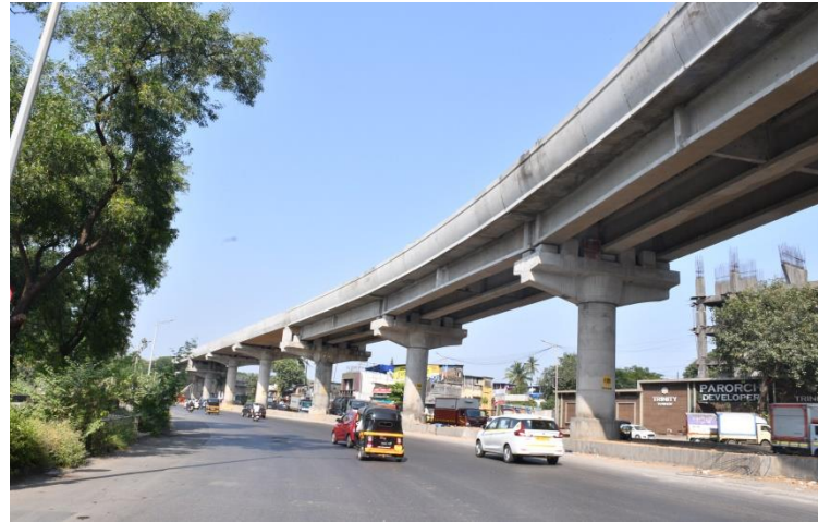
Mumbai Metro Line 6
