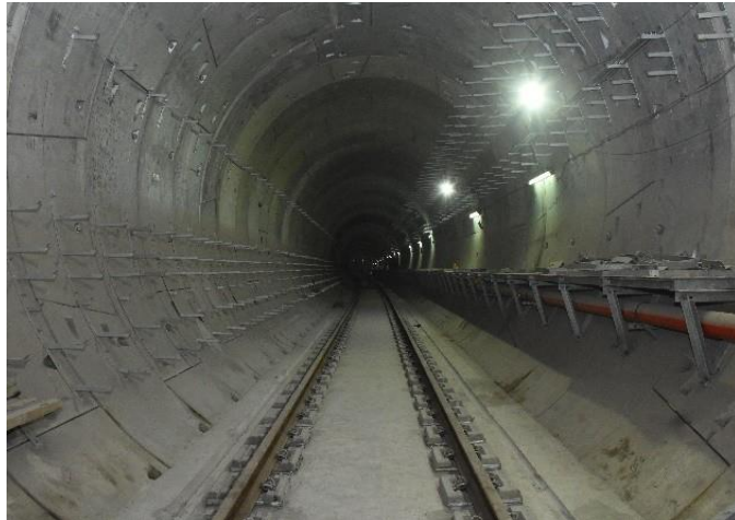
Mumbai Underground Metro Line 3
