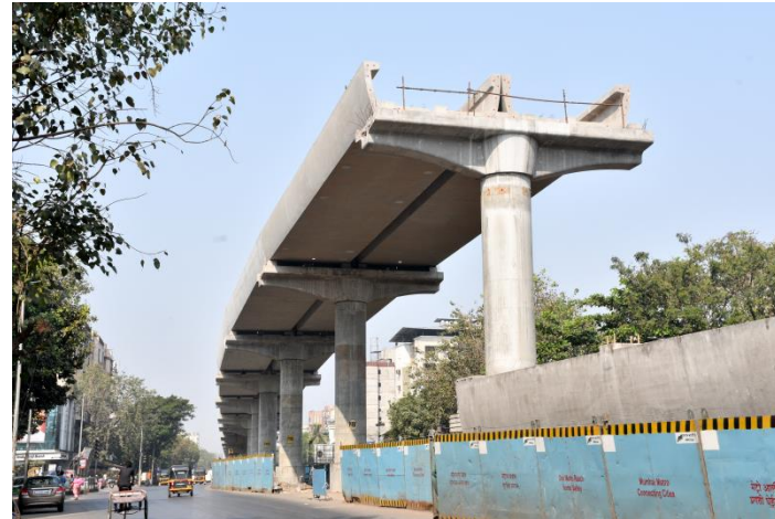
Mumbai Metro Line 9
