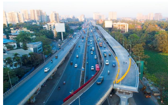
Chheda Nagar Flyover Part 1
