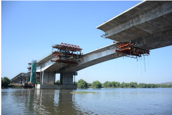
Motagaon Creek Bridge
