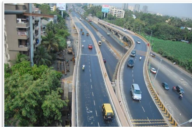
Amar Mahal Flyover
