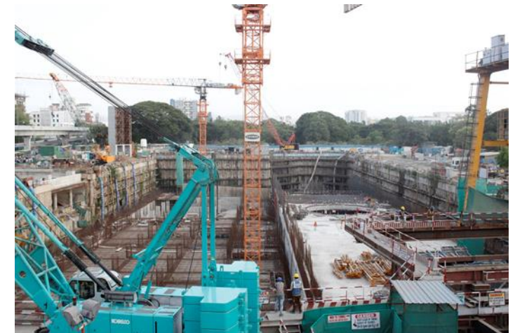
Pune Underground Metro
