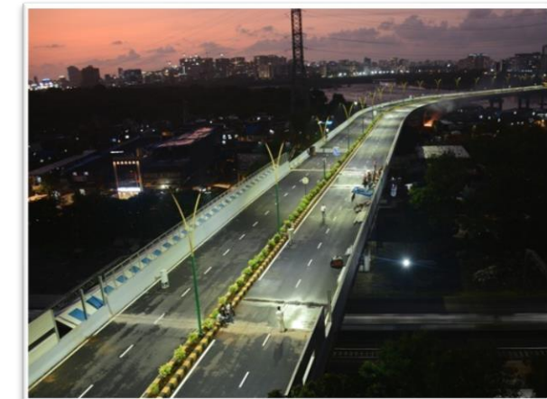
BKC- Chunabhathi Flyover
