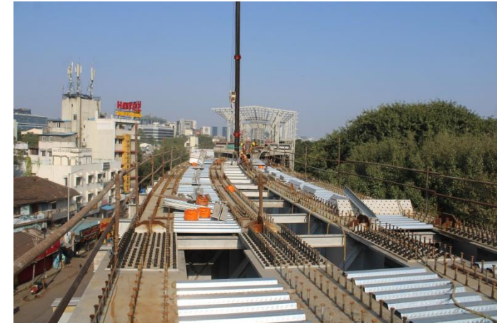
Pune Elevated Metro
