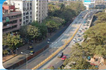
Flyover at Hindmata
