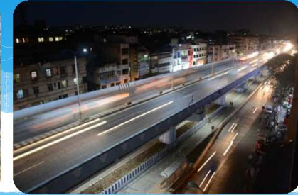
Flyover at Dhanakwadi
