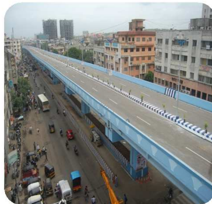
Dhankawadi Flyover, Pune
