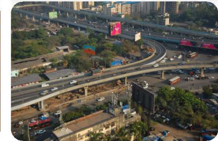
Flyover at Kapurbawadi
