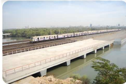
Bridge at Bandra -Mahim
