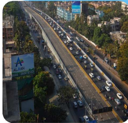
Kherwadi Flyover, Mumbai
