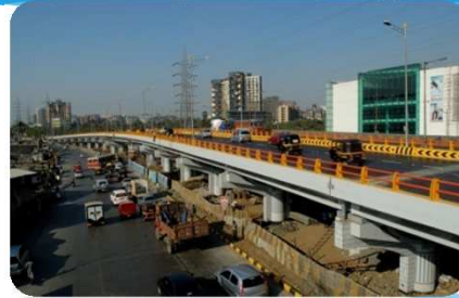
Flyover at Dindoshi, Mumbai
