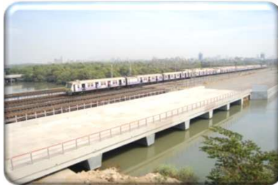
Bridge at Bandra -Mahim
