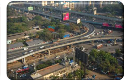
Flyover at Kapurbawadi
