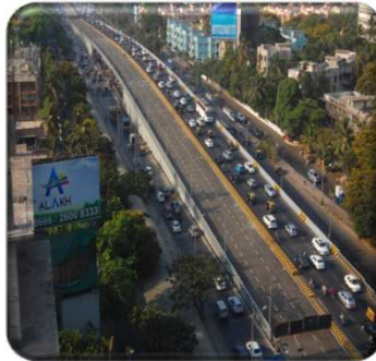
Kherwadi Flyover, Mumbai
