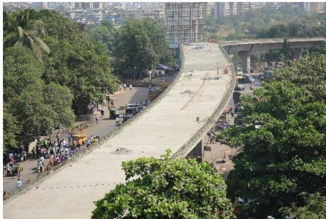
Kalwa Bridge Thane
