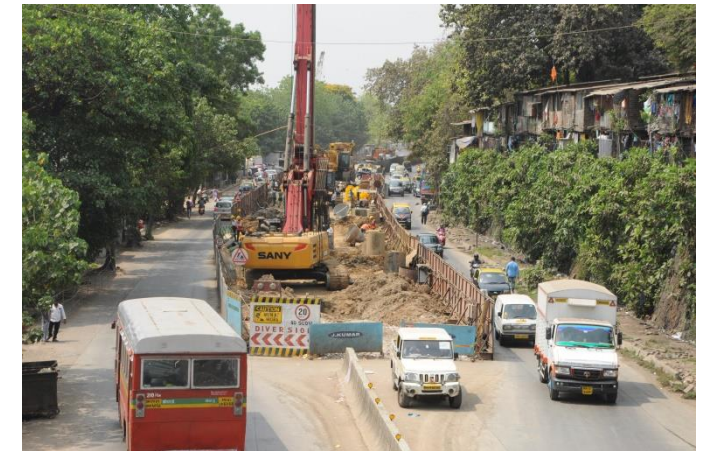
Sewri Worli Elevated
