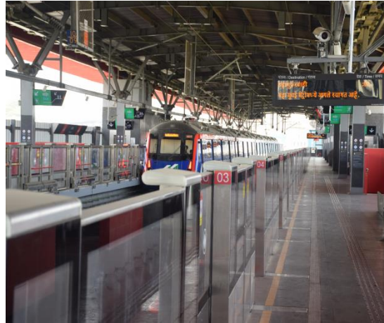
Mumbai Metro Line 7
