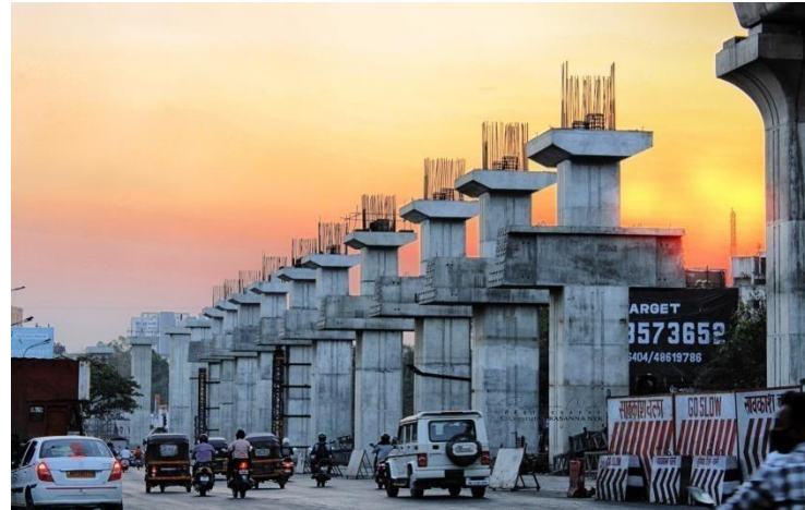
Pune Elevated Metro
