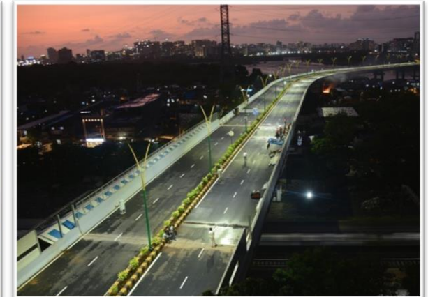
BKC- Chunabhatti Flyover
