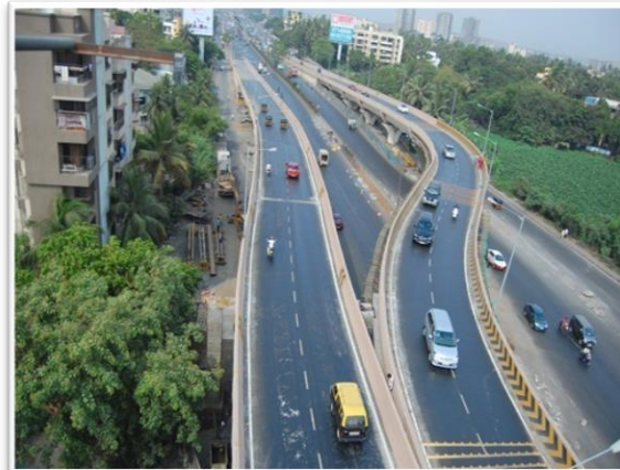
Amar Mahal Flyover
