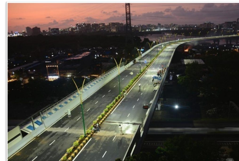
BKC- Chunabhatti Flyover
