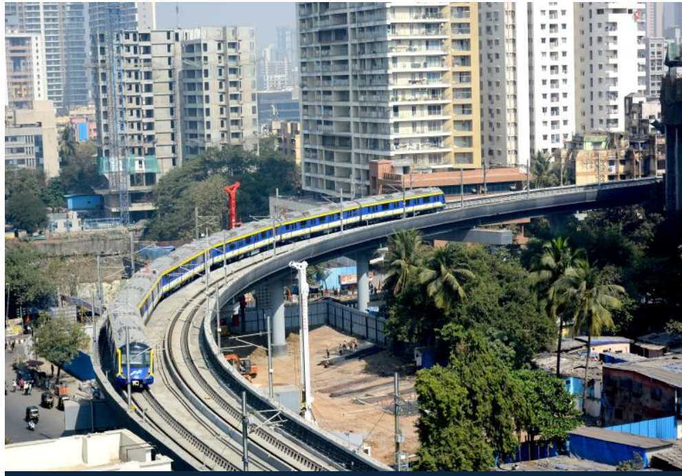
Mumbai Metro Line 2A
