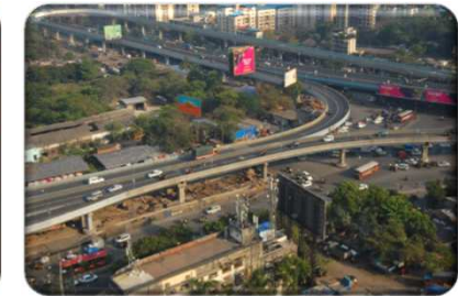
Flyover at Kapurbawadi
