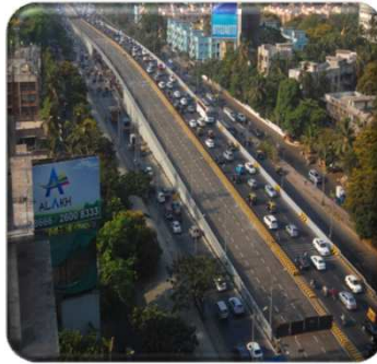
Kherwadi Flyover, Mumbai
