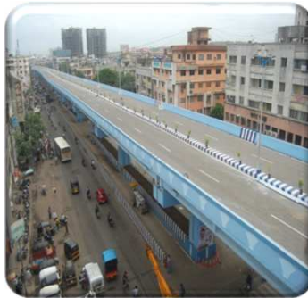
Dhankawadi Flyover, Pune
