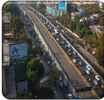
Kherwadi Flyover, Mumbai
