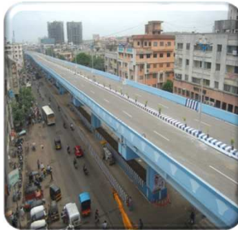
Dhankawadi Flyover, Pune
