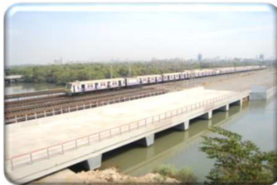
Bridge at Bandra -Mahim
