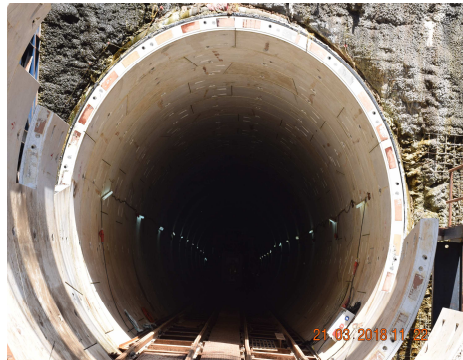
Mumbai Metro Line - 03
