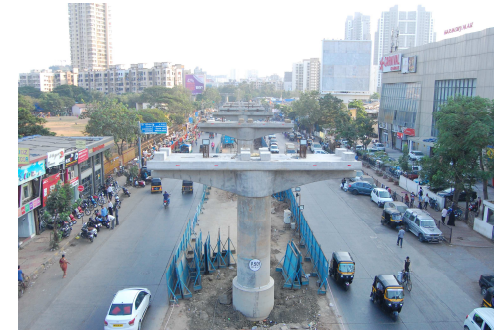
Mumbai Metro Line - 02
