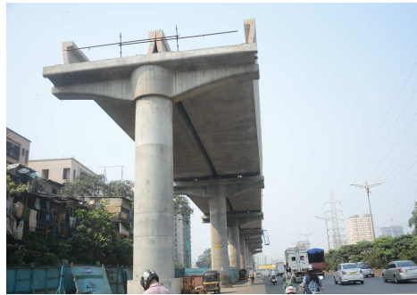
Mumbai Metro Line - 07
