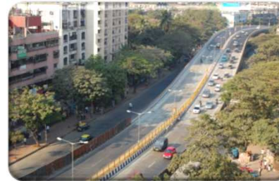
Flyover at Hindmata
