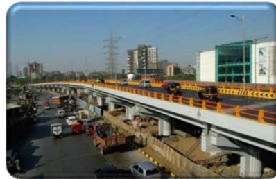
Flyover at Dindoshi, Mumbai
