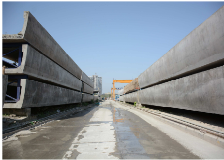
Bandra Casting Yard MML-07
