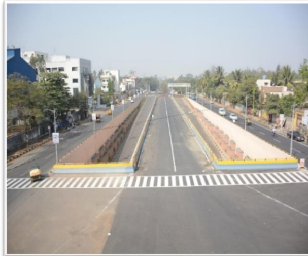
KSB Underpass, Pune
