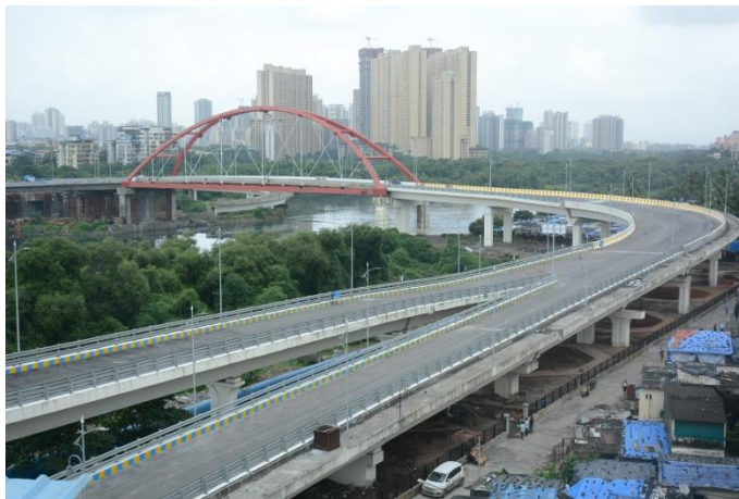
Kalwa Bridge Thane
