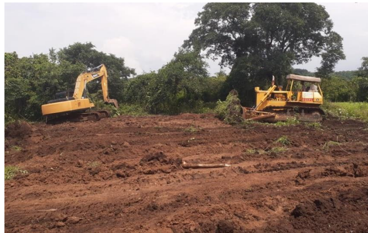
Vadodara Mumbai Expressway, IRCON
