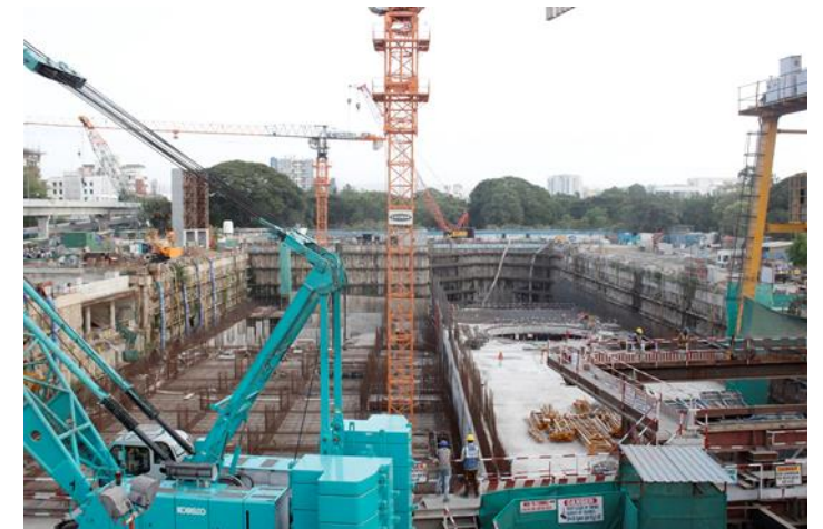
Pune Underground Metro
