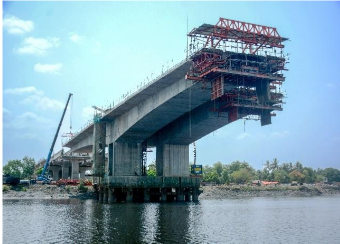
Motagaon Creek Bridge
