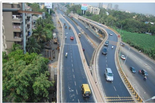
Amar Mahal Flyover
