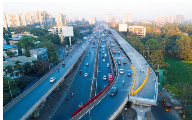
Chheda Nagar Flyover Part 1
