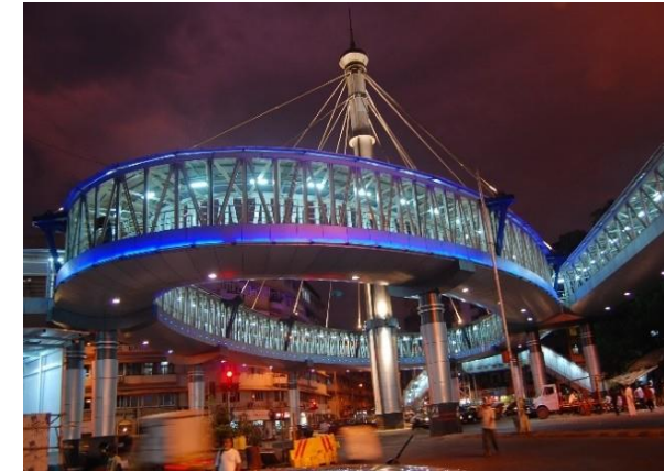
Grant road Skywalk
