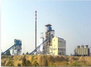
10 MW POWER PLANT FOR VARUN BIO ENERGY
