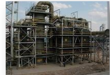
GAS CLEANING PLANT FOR KCM, ZAMBIA
