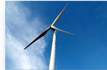
1.5 MW WIND TURBINE AT UTHUMALAI
