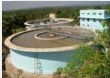
WATER TREATMENT FOR TWAD BOARD
