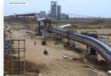
CROSS COUNTRY CONVEYOR FOR SREE JAYAJYOTHI CEMENT
