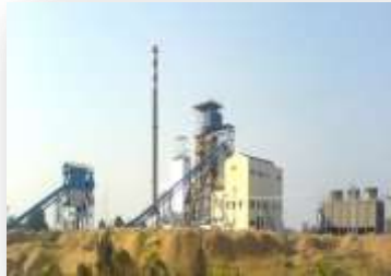
10 MW POWER PLANT FOR VARUN BIO ENERGY
